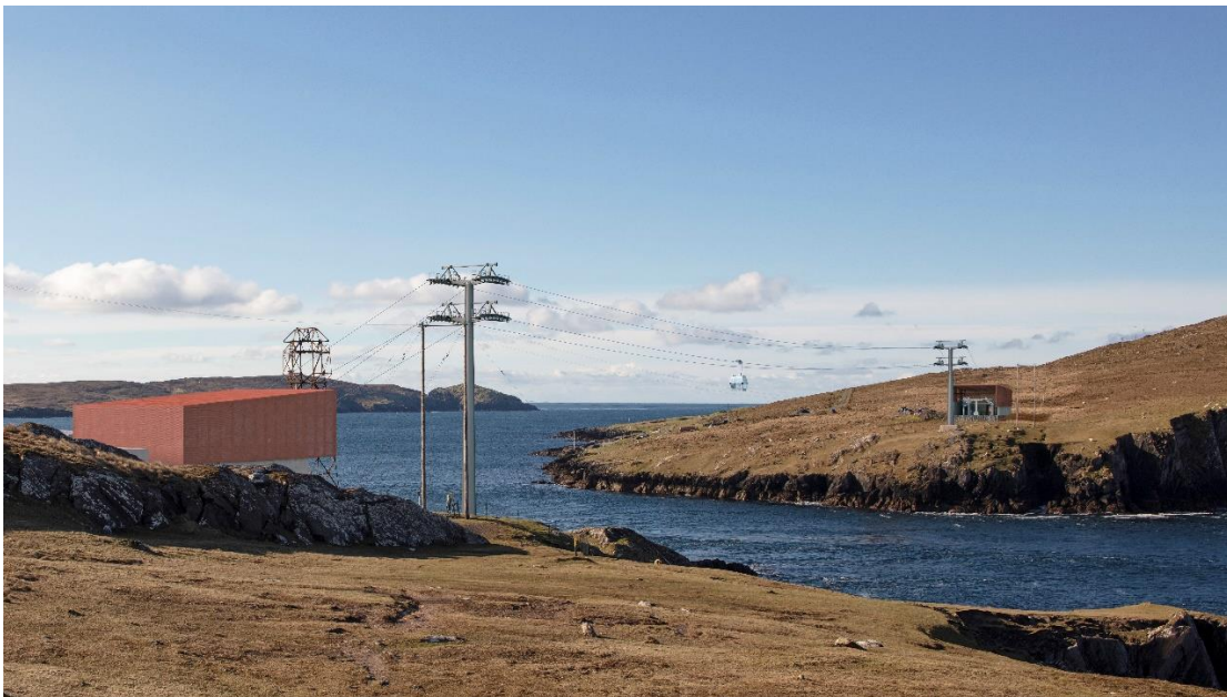
Plate 4.29 Artists impression of the mainland line station (with island line station in the distance) as seen from the north.
